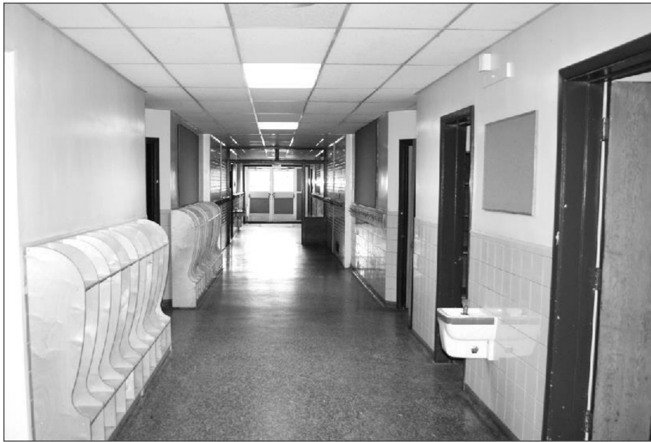
Now that school is out for the summer, the hallway and classrooms of the old wing at DYS have been cleaned out and emptied. Students returning to school in the fall will be able to make use of the new wing's upgraded classrooms, accessibility features, and expanded playground behind it.
